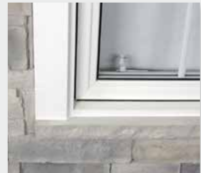
Finish with window sill, trim and jamb
